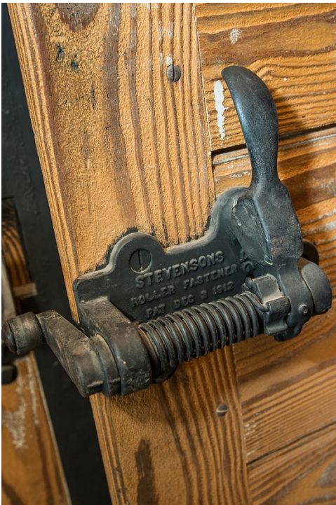
Photo 22 Second floor cold storage door, Stevensons hardware, original, typical throughout
