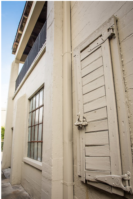
Photo 6 Original door and hardware, north elevation
